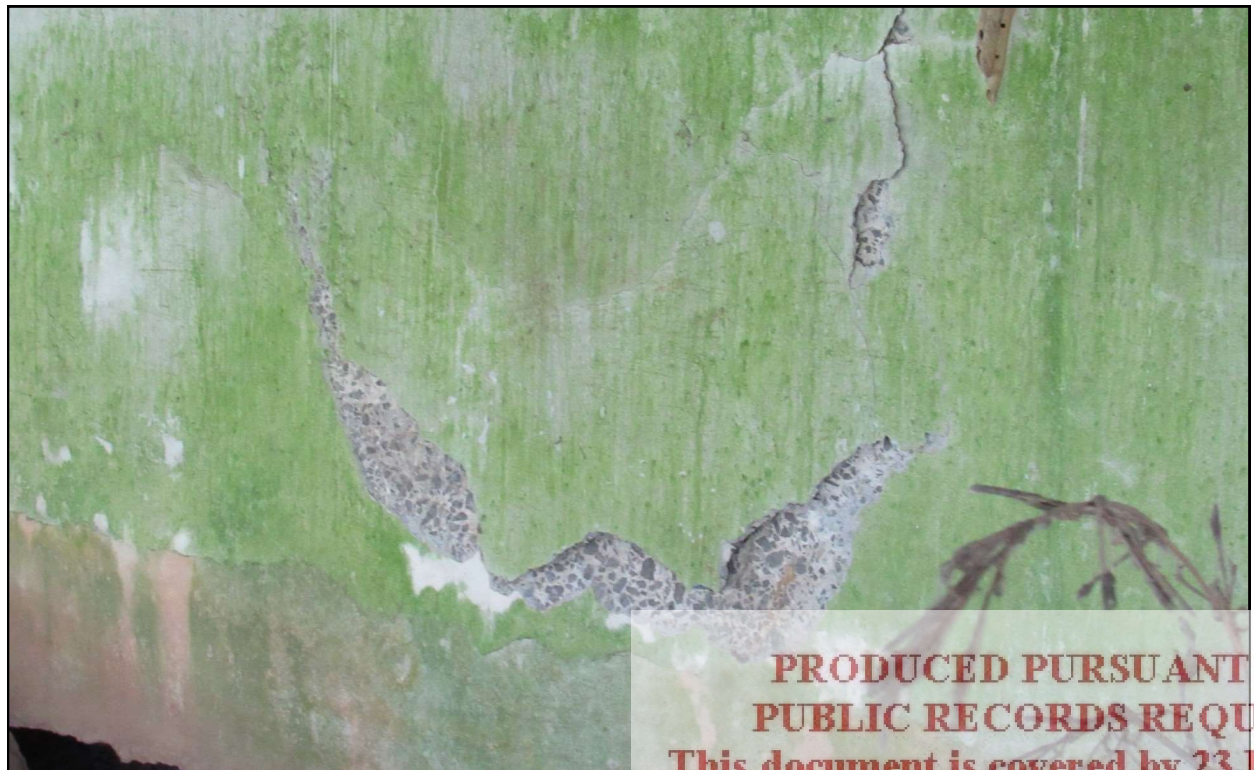
DELAM AT ABUTMENT #2
